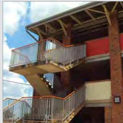
New classrooms at Buyani Primary School
