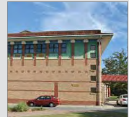
Refurbished Fort Hare National Archives
